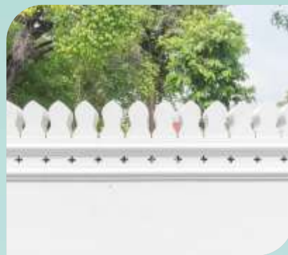
5FT. HIGH COMPOUND WALLS
